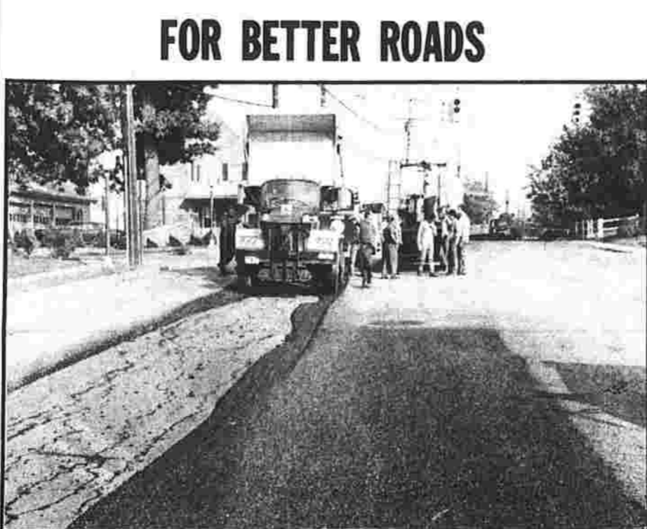
Repaving of E. Middle Turnpike Nearing Completion
